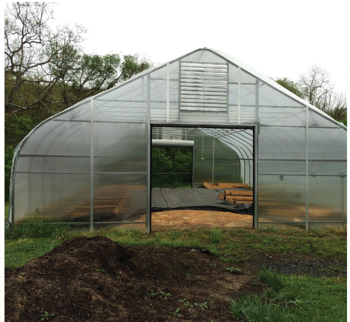
Newly Constructed High Tunnel in Romney WV
